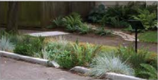
Planting Strip Trench
